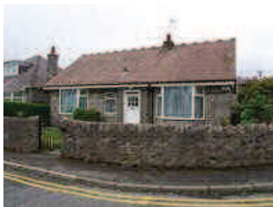
The existing house and site from North
